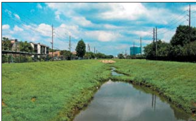
Unimproved drainage canal
