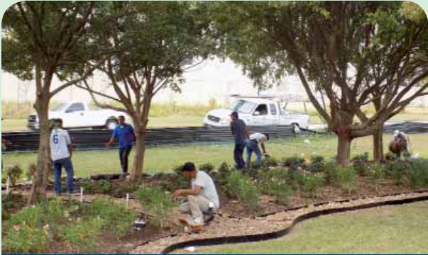
Preventing a washout: The southbound greenspace between the West Sam Houston Tollway and Beltway 8 just north of Westheimer becomes more erosion resistant with strategic plantings.
