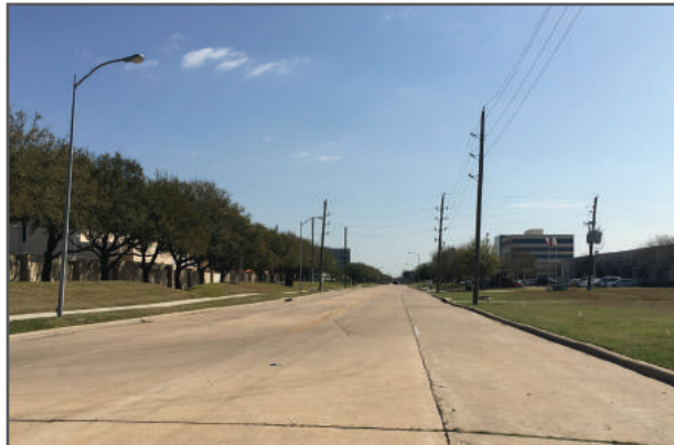
eastbound at utility easement
