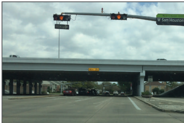
eastbound at Beltway 8
