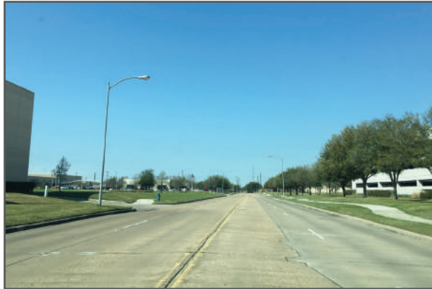
westbound near Rogerdale Lane
